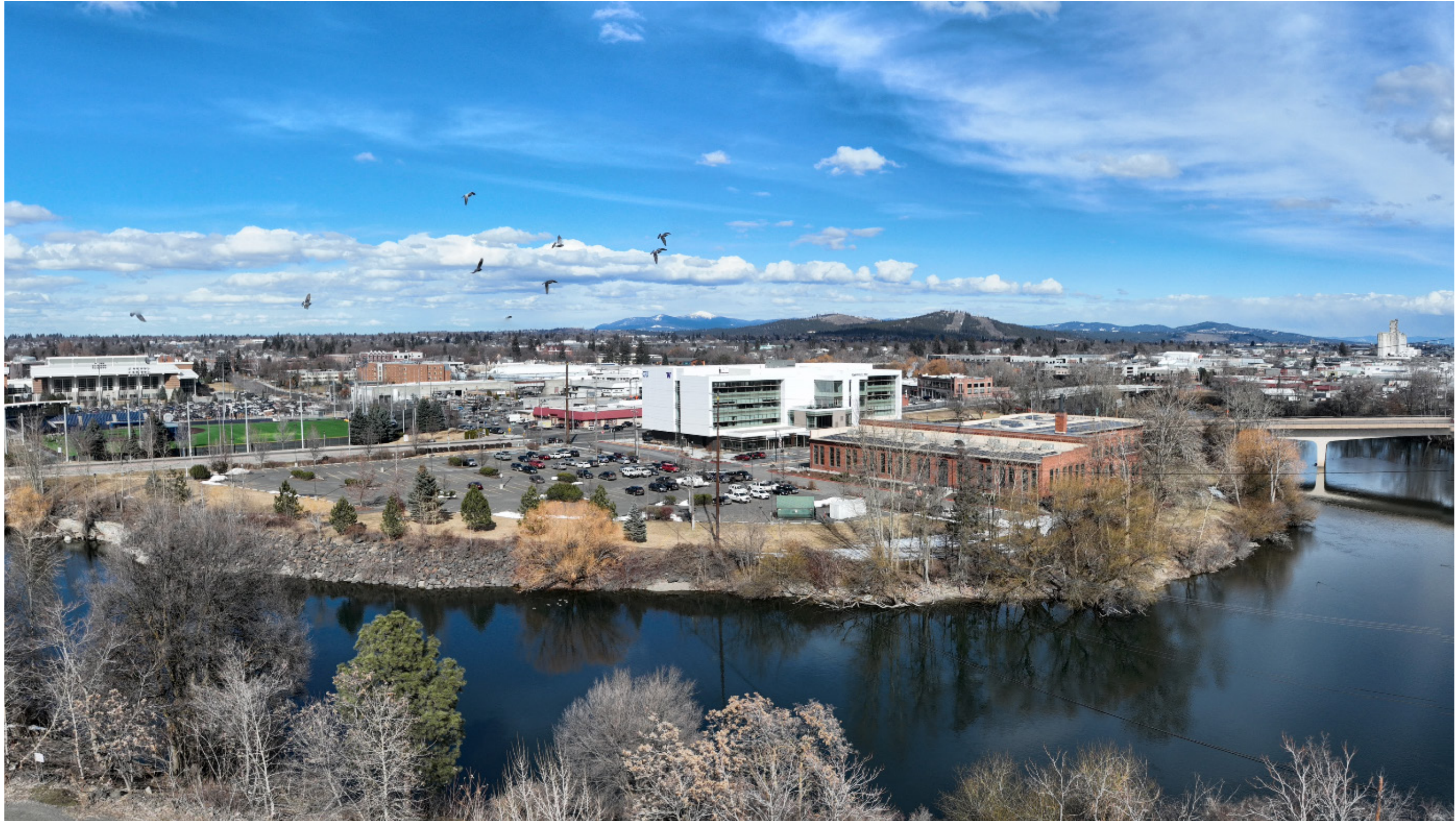
DRONE PHOTO - 68' ELEVATION
