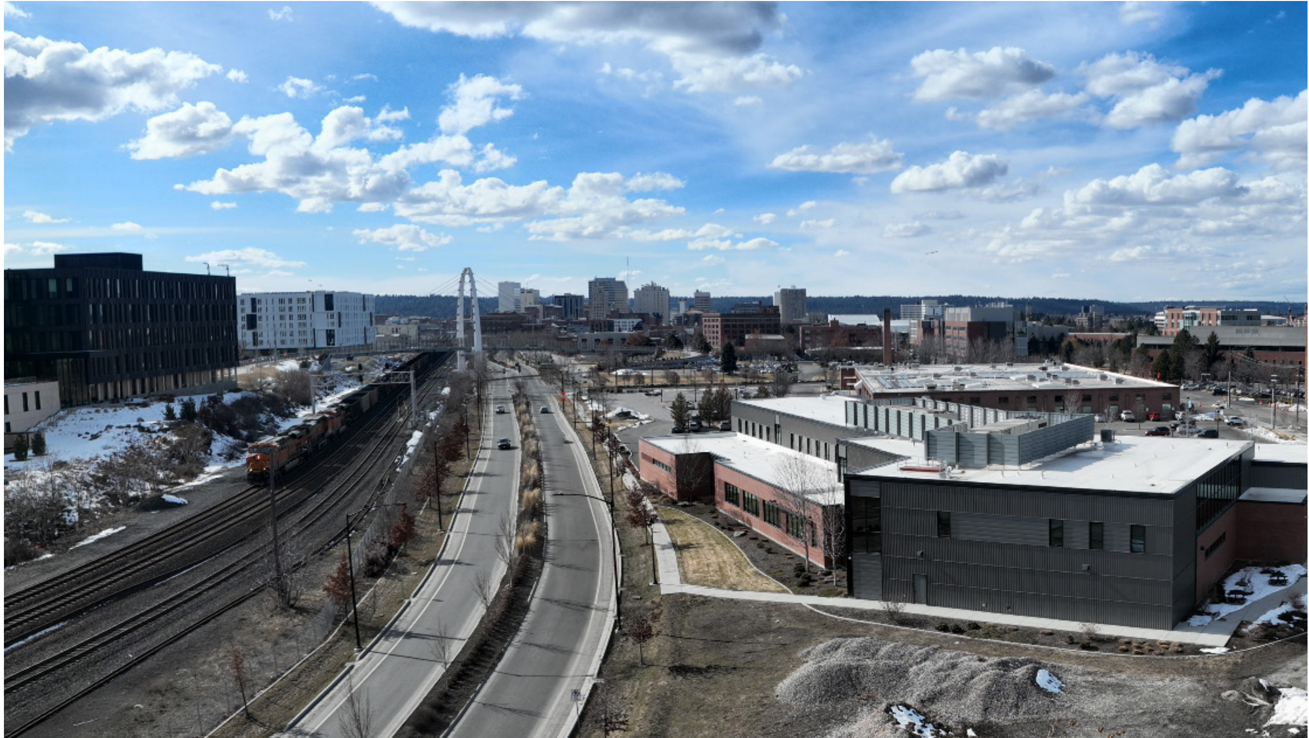
DRONE PHOTO - 68' ELEVATION
