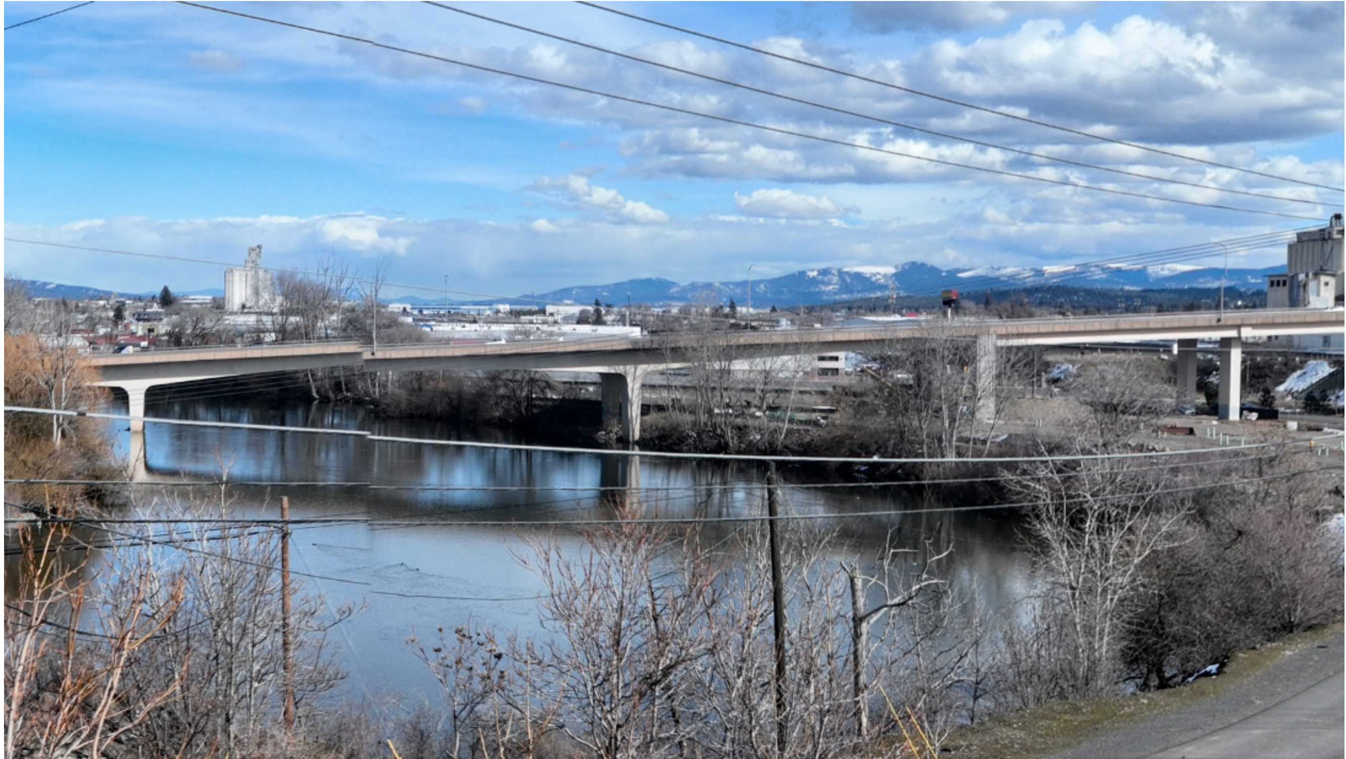
DRONE PHOTO - 20' ELEVATION
